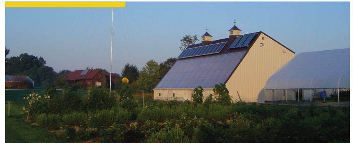
Barry Adler's BioIntegrated Greenhouse (left) is powered by a wind turbine and solar array, and is heated with a solar radiant floor system; the Passive Solar Greenhouse (right) has no supplemental heating.
