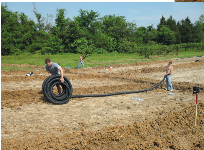
Before planting a peach orchard in an area with wet clay soil, Barry Shortt and crew installed a do-it-yourself drainage system to improve tree survival and vigor.
