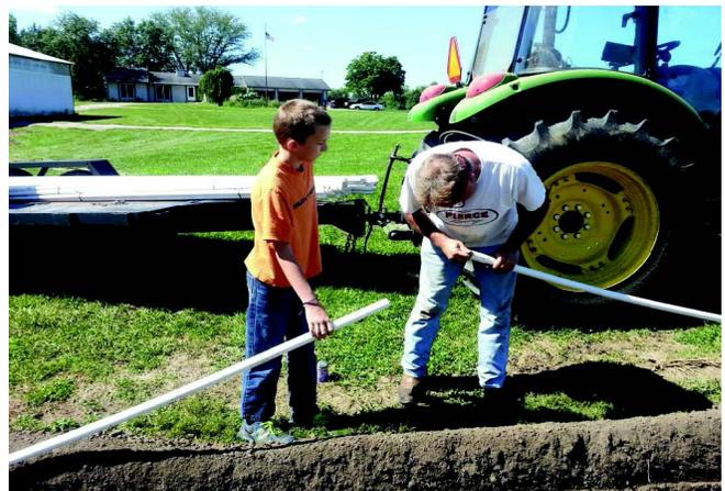
With sprinklers, lasers, sensors, timers, electronic water valves, and 1,700 feet of PVC pipe, Cary's You-Pick Farm in Kearney, Missouri, devised a sprinkler deterrent system which has greatly reduced racoon and deer pressure.
